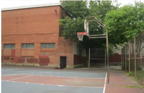
North Building Façade
