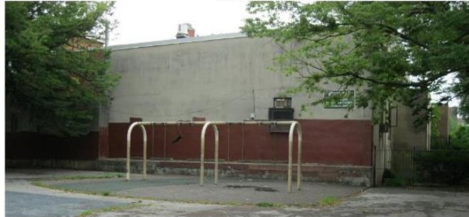
North Building Façade
