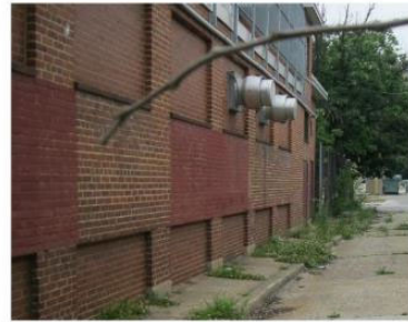
East Building Façade
