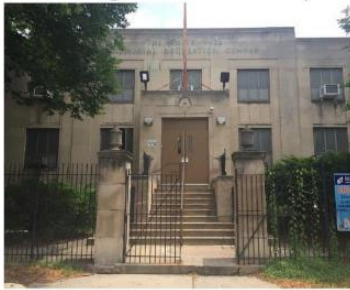
West Building Façade
