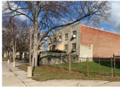
South Building Façade
