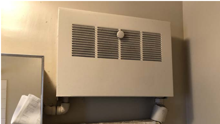
TYPICAL WALL-MOUNTED RADIATOR
