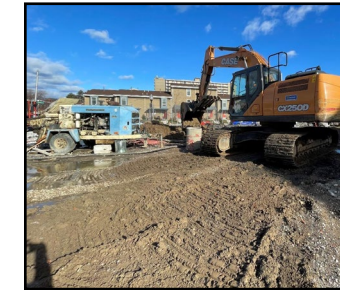
P&J workers cleaning and grabbing the jobsite.
