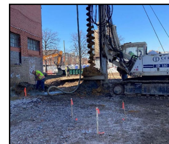
Pumping grout into the pile.
