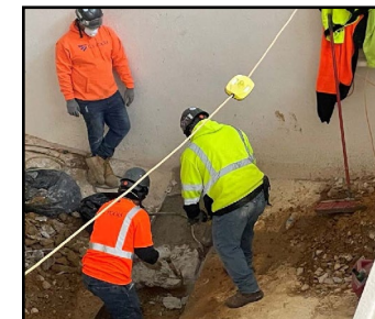
US Pools jackhammer, saw, and cut the existing pool drainpipe.
