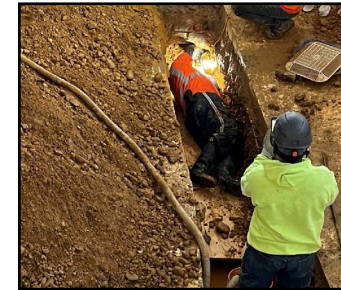
US Pools continue to work on the existing pool.
