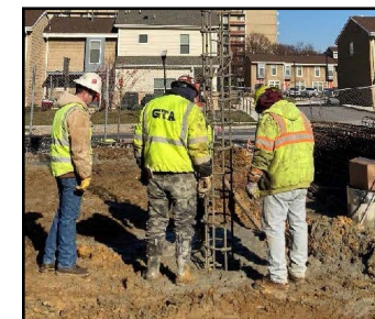
Lowering the steel rebar cage into the ground.
