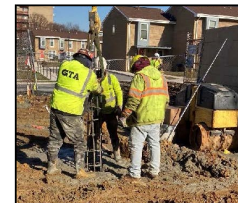
Lowering the steel rebar cage into the pile.
