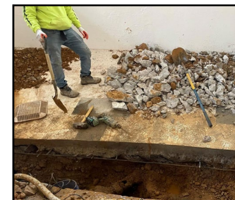
US Pools saw cutting the existing pool floor.
