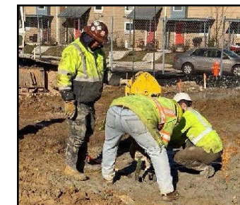
Inserting the steel rebar cage into the pile.
