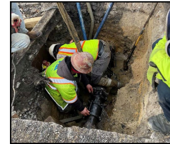
Harrington workers install a 6" water valve.
