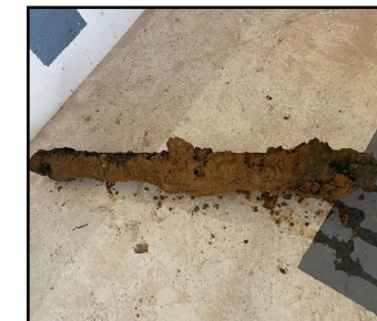
US Pools remove the existing pool drainpipe.
