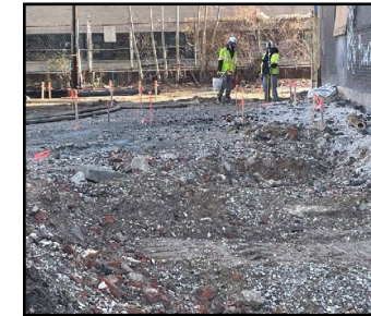
Dewberry workers setup elevation for pile & footing.
